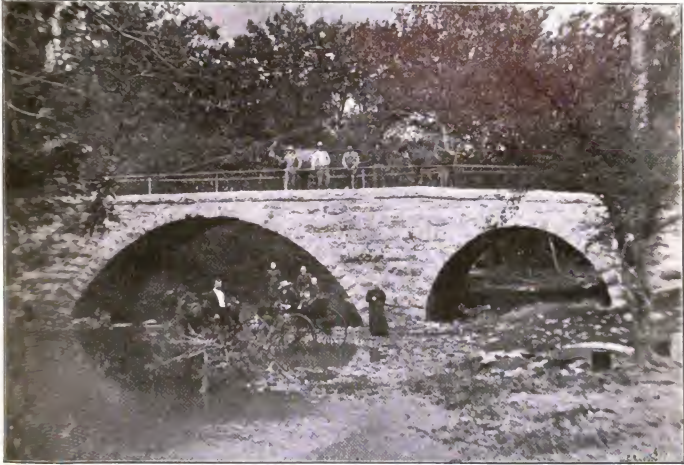
NORTH MAIN STREET BRIDGE, EL DORADO, KANS.
